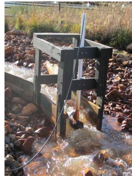
New water turbine at Tanoma installed Fall 2013
